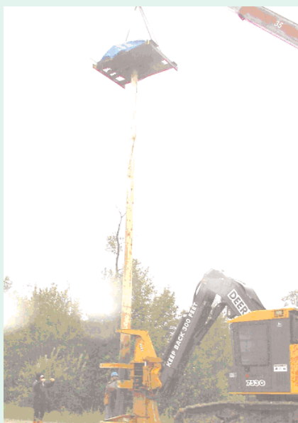
Crane placing pole in feller/buncher for move to new location
